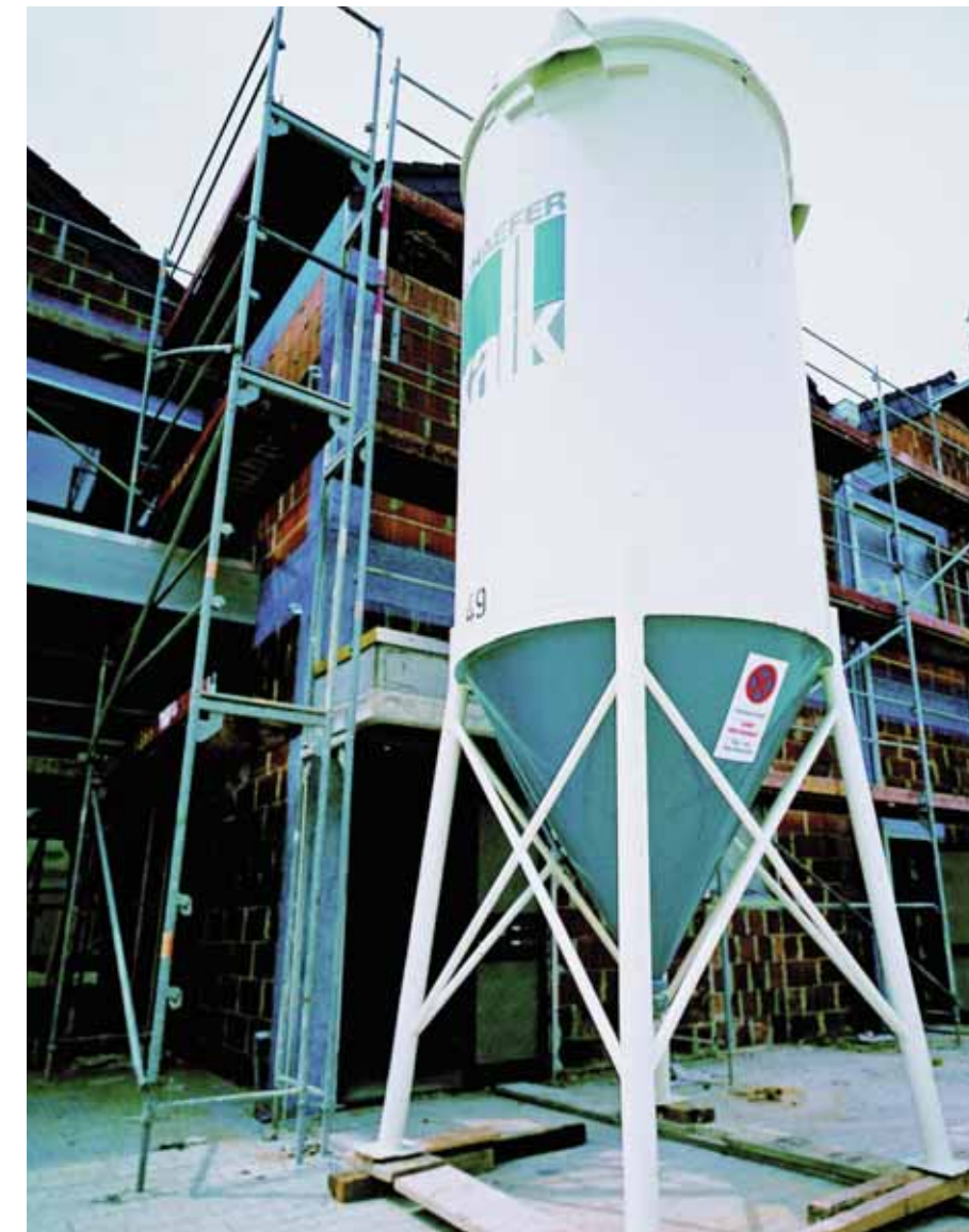
Baustellensilo Trockenmörtel Construction site silo for dry mortar
