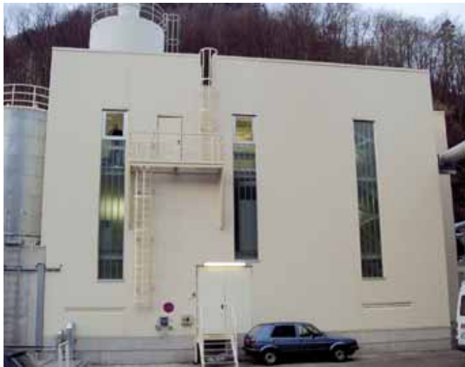
PCC-on-site-Anlagen: links Neidenfels, rechts Wattens PCC on-site unit: left Neidenfels, right Wattens
