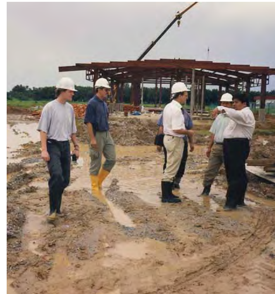
Baustelle in Malaysia, 1996 Construction site in Malaysia, 1996
