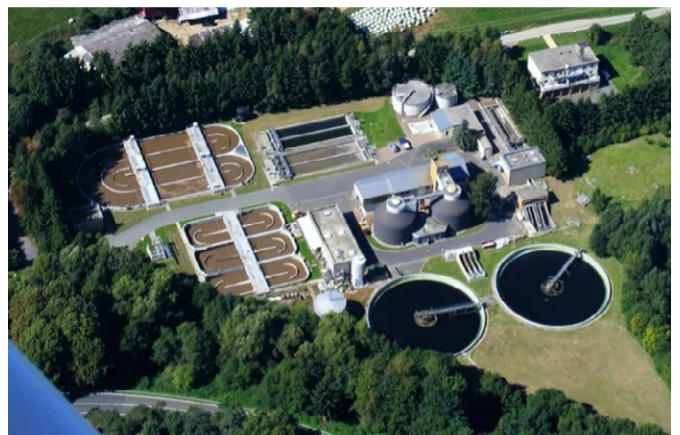
Fig. 1: Wastewater treatment plant Bleidenstadt
